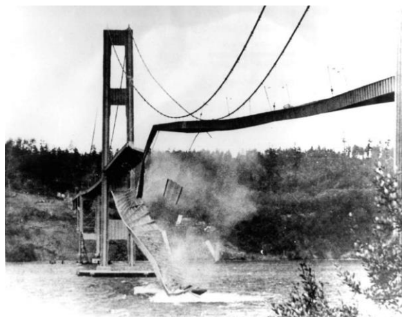
Figure 6. New Tacoma Narrows center span crashes into Puget Sound, November 7, 1940, www.seattlepi.com
