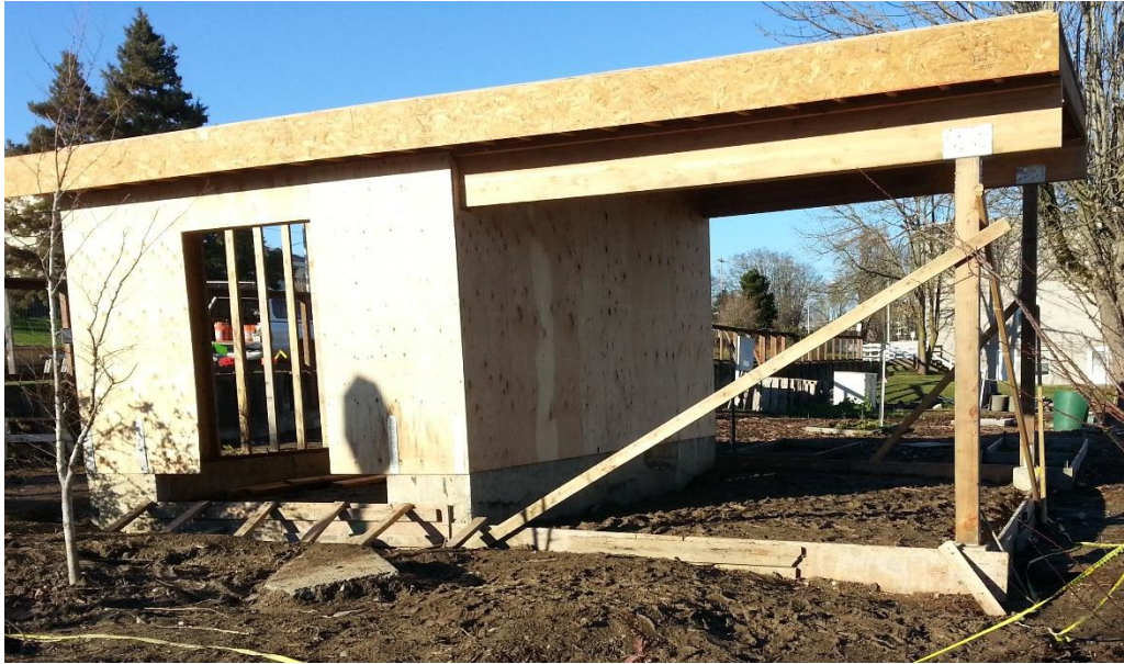
Figure 8: The East straw bale wall after plywood sheathing
