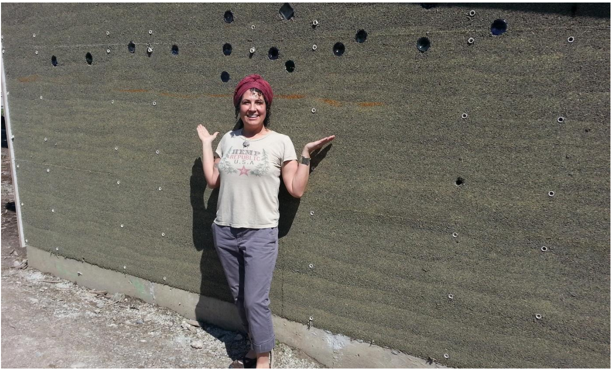
Figure 9: Joy Beckerman of Hemp Ace Technologies in front of the SHED's hemp-lime wall
