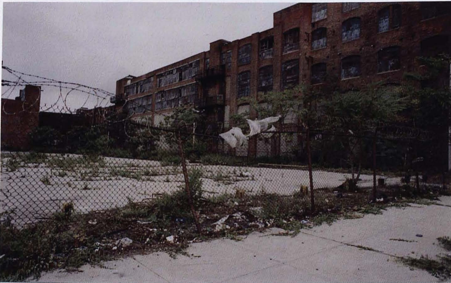
Abandoned Building on East River in Williamsburg, Brooklyn
